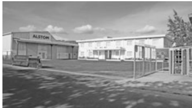
New reconditioning facility in Phu My (Vietnam).
