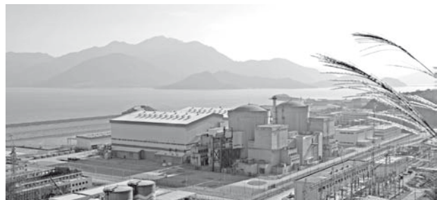
Ling Ao Ph 1 & 2, China nuclear power plants using ARABELLE™ steam turbine and generator.
